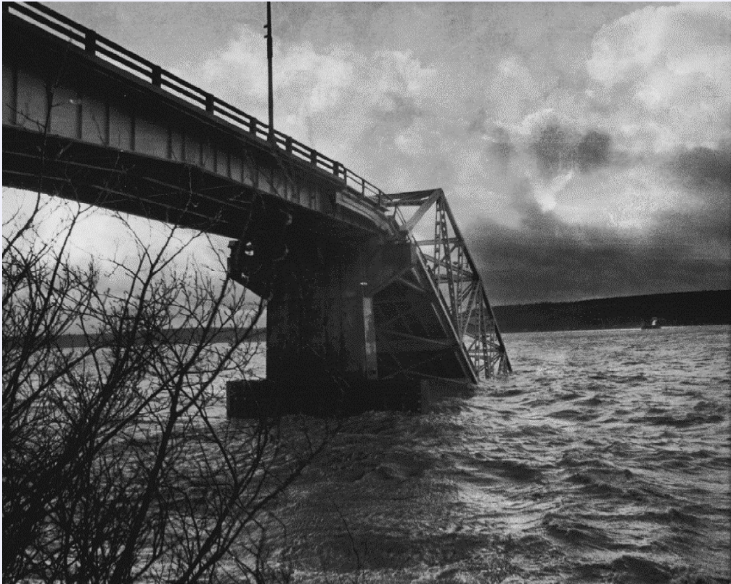
Feb. 13, 1979: Winds over 100 kts destroyed the Hood Canal Bridge Cost to replace: over 100 million dollars
